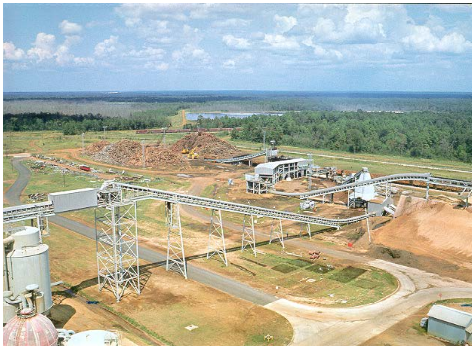
Figure 3. Raw Material Handling Area Showing Log Piles, Debarker, Chipper, Chip Piles and Conveyors.
