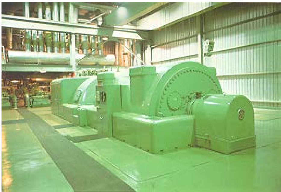
Figure 15. Steam Turbine-Generator
